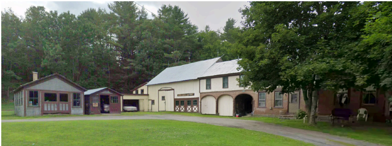
H3 Batchelder Plumbing & Heating 110 Mill St Plainfield
